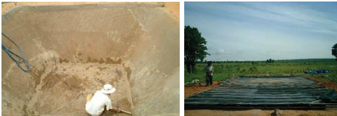
Figure 5.7 Rainwater harvesting with sand-cement storage pond in Vietnam
